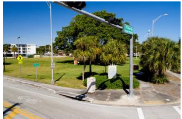
Utility Box Aerial View
